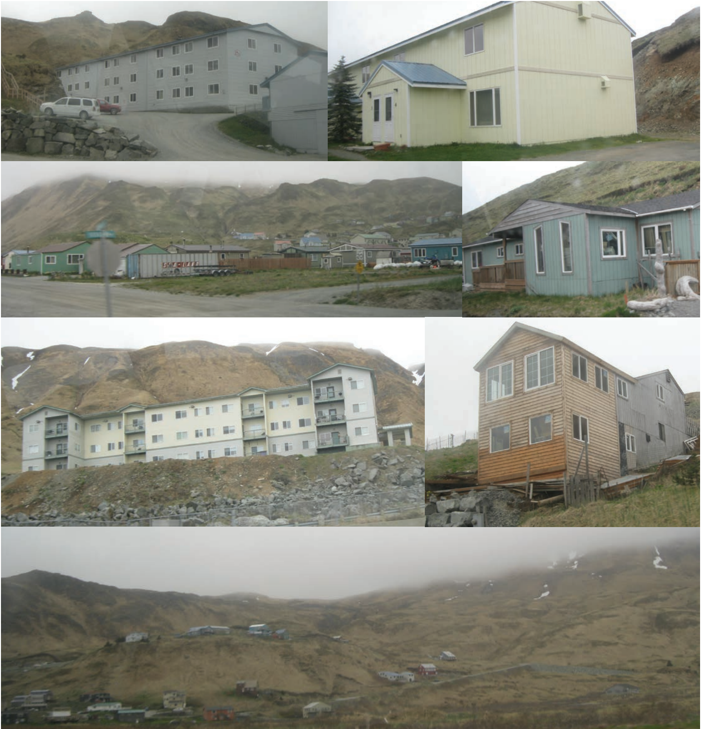
Images 23-29: Photographs of different housing stock and a demonstration of the building challenges related to the topography in Unalaska. Photos by Ryan Scherzinger
