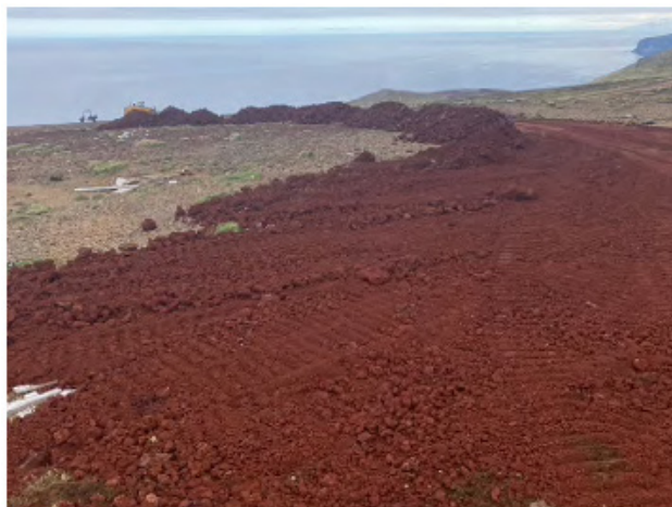
Description: Capping material staged along eastern edge of SS002 (facing northeast). (6/14/2021)
