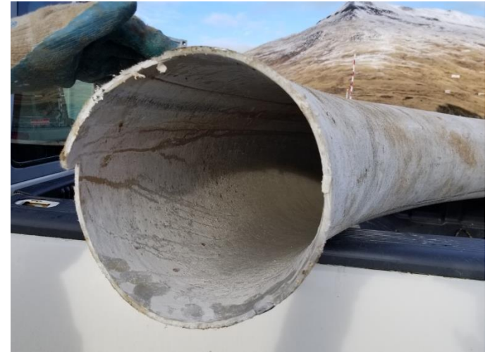
Excess Slip-Lining Material After Curing
