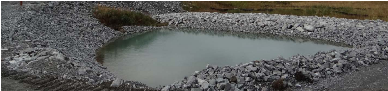
Photo 6-2. Sediment Basin at Ugadega Quarry
