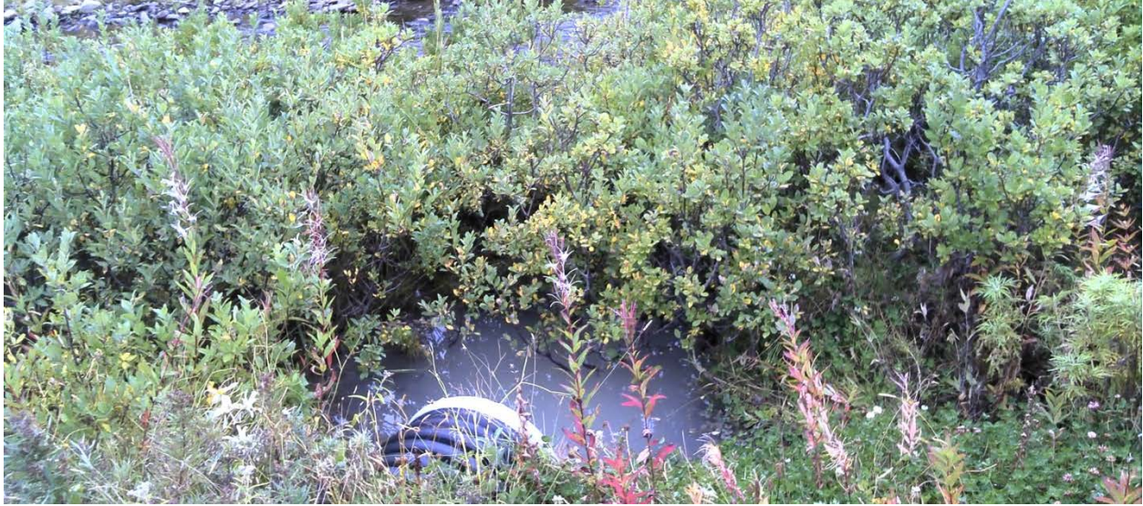
Photo 8-2. Sediment-Laden Stormwater Discharge
