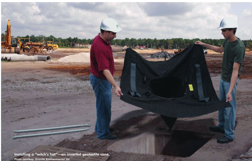
Figure 6-1. Witch's Hat Installation (Williams-Villano 2013)
