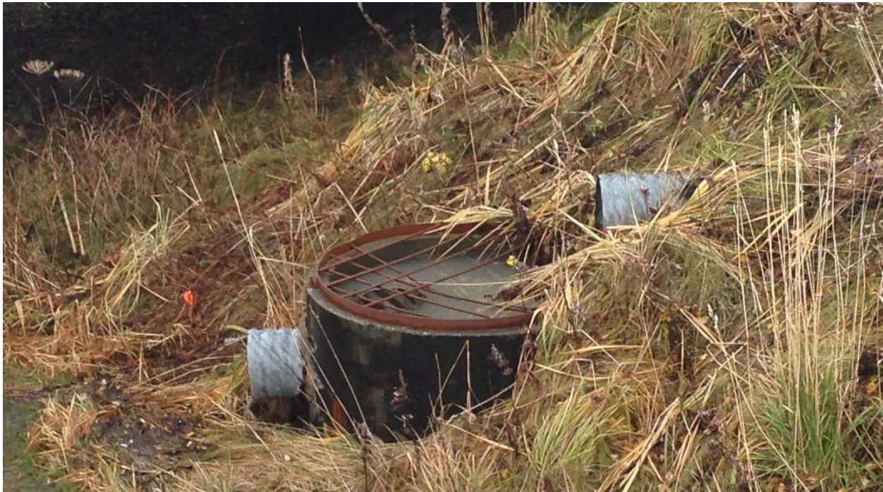
Photo 8-5. Engineered Outfall at 5th Street Bridge
