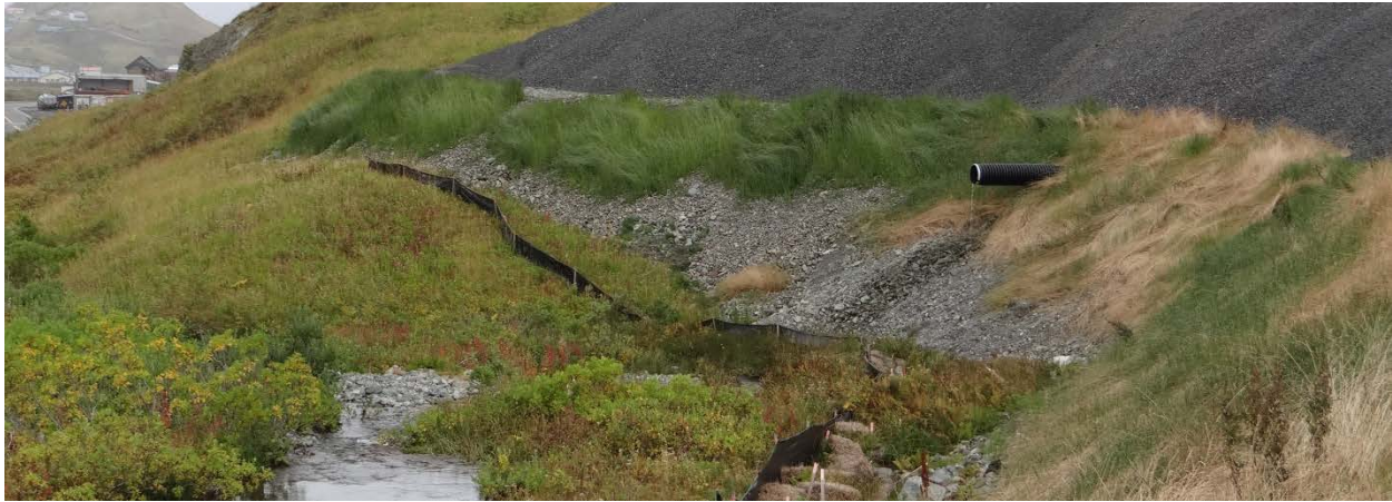
Photo 6-1. Silt Fence, Straw Wattles, and Seeded Slopes in Use at City Stockpile
