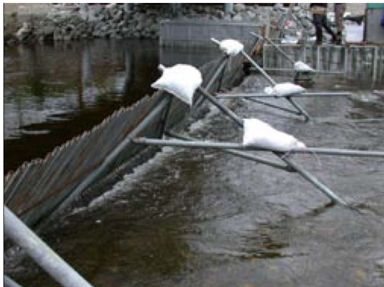
Photo 3-4. Rigid Tripod Weir Example (Zimmerman & Zabkar)
