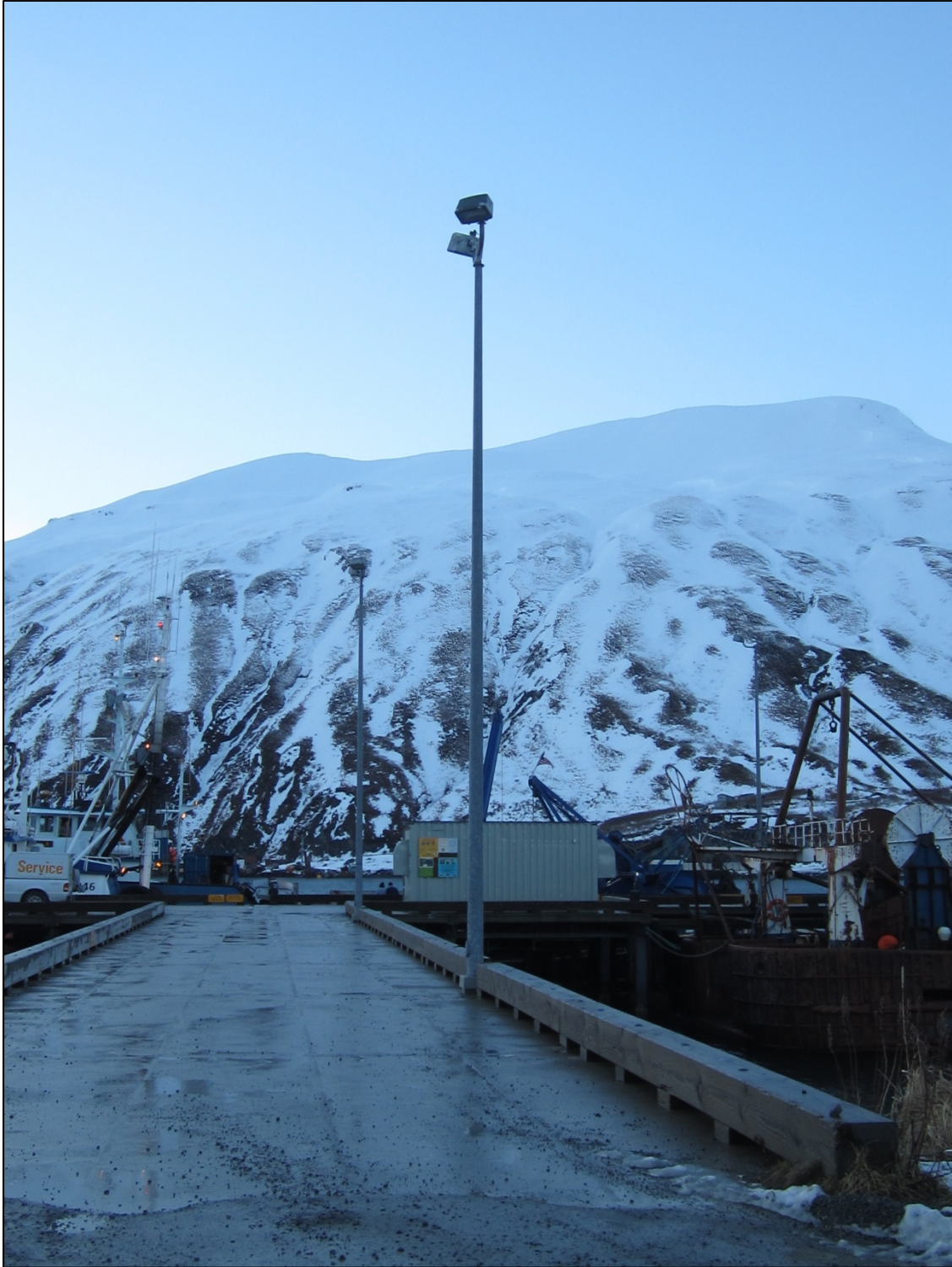
PHOTO 13. Light Pole on Approach at Spit Dock.
