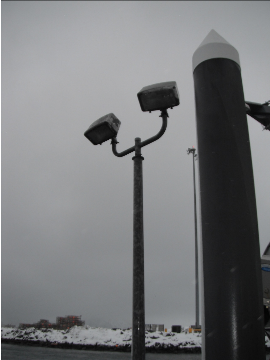
PHOTO 14. Light Pole on Floating Dock at Spit Dock.
