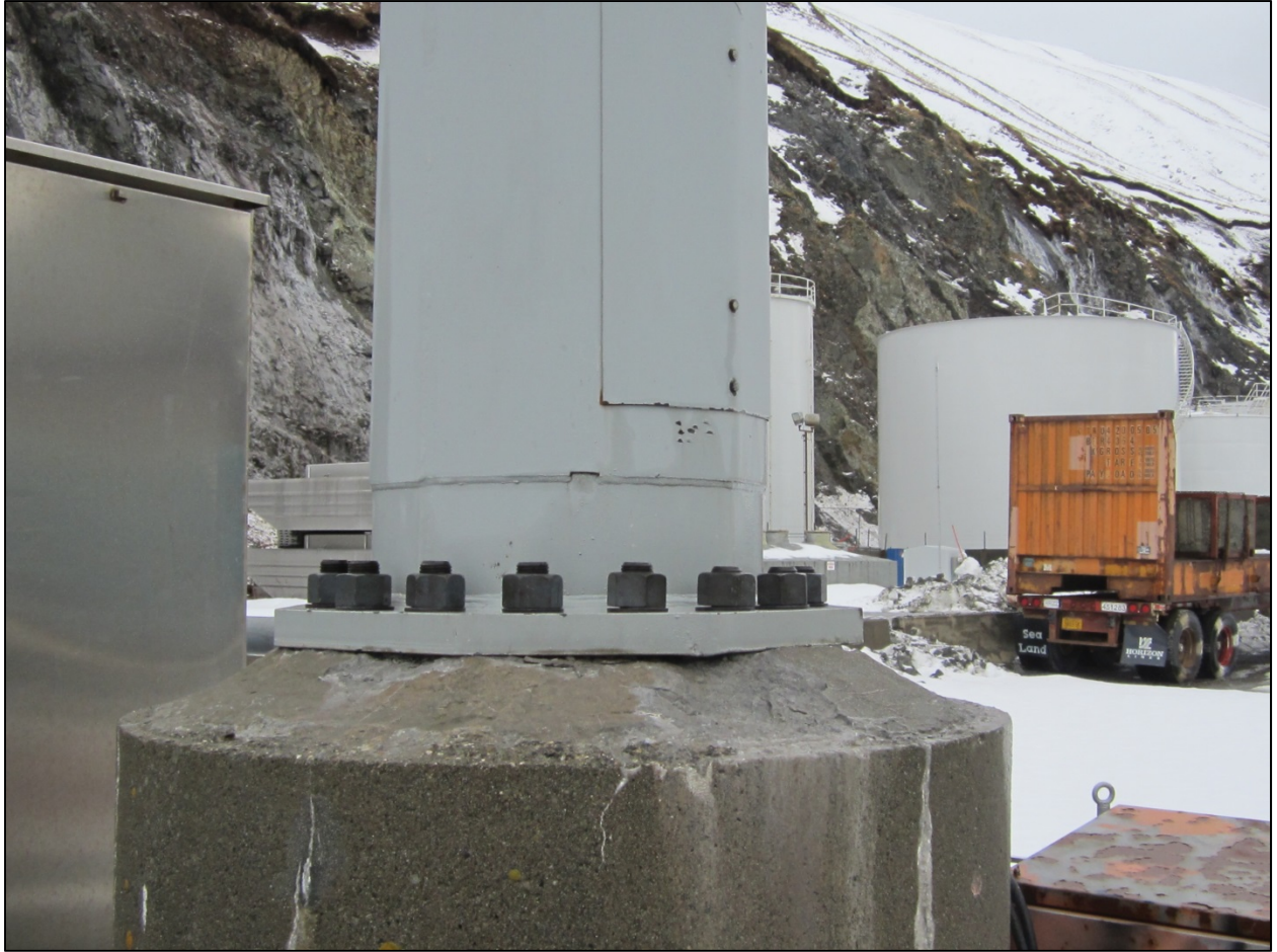
PHOTO 3. Base of South HML at UMC City Dock.
