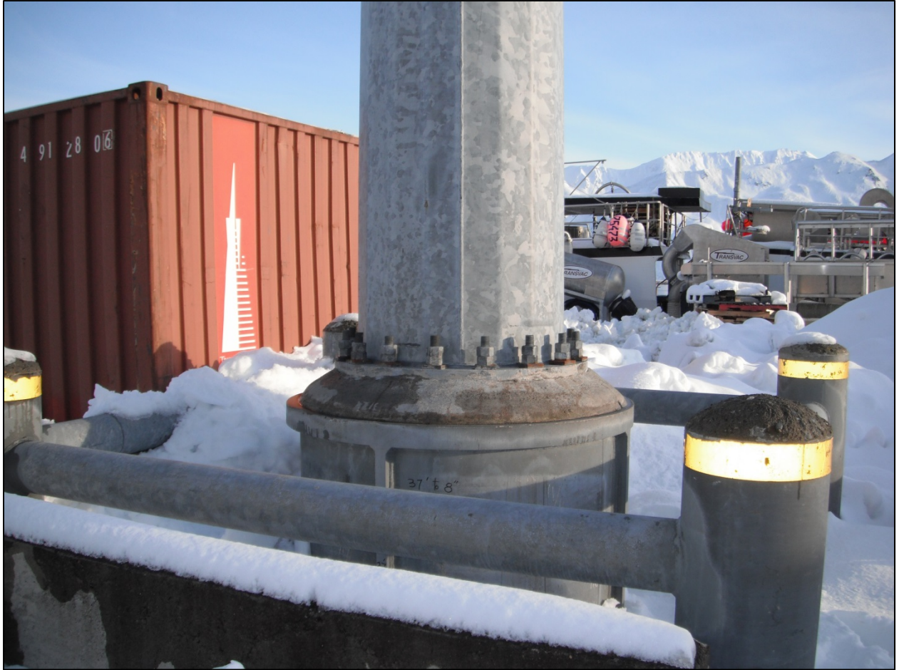
PHOTO 6. Base of South HML at UMC USCG Dock.
