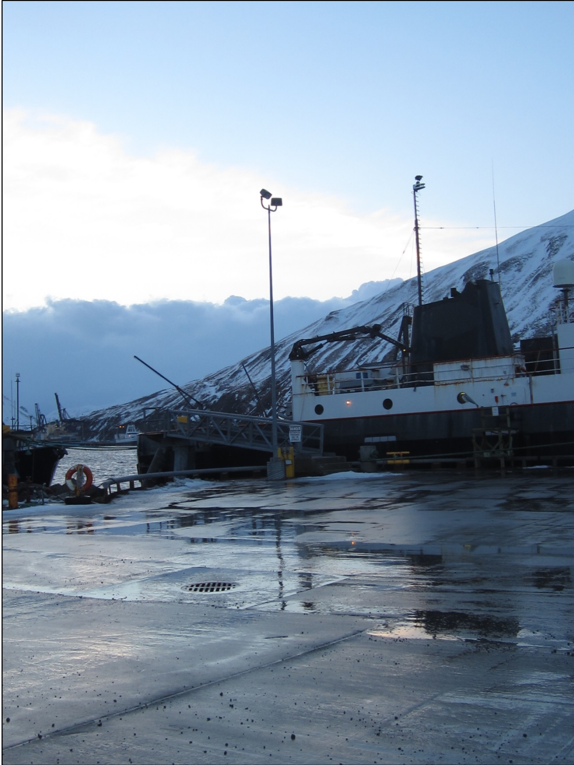
PHOTO 10. Light Pole at Light Cargo Dock.
