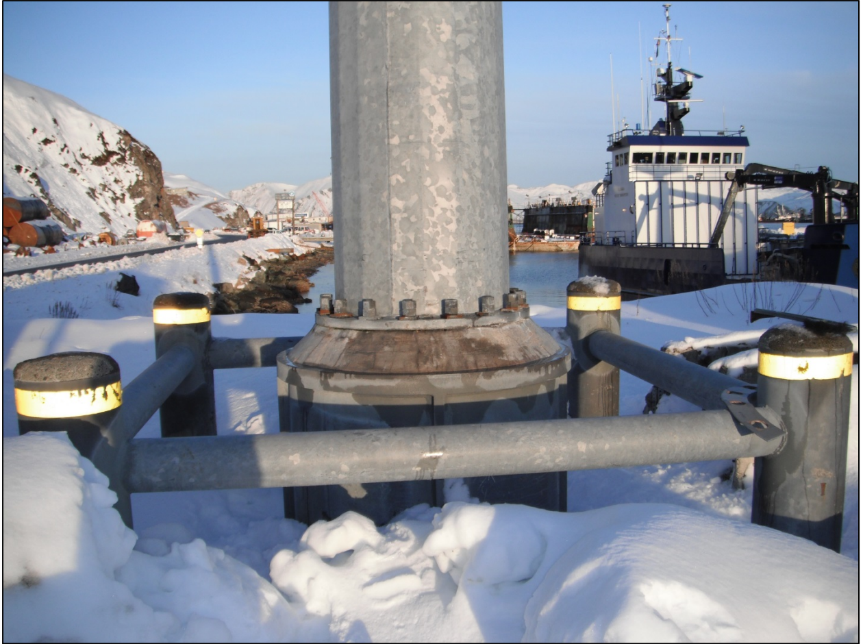
PHOTO 7. Base of North HML at UMC USCG Dock (looking NE).
