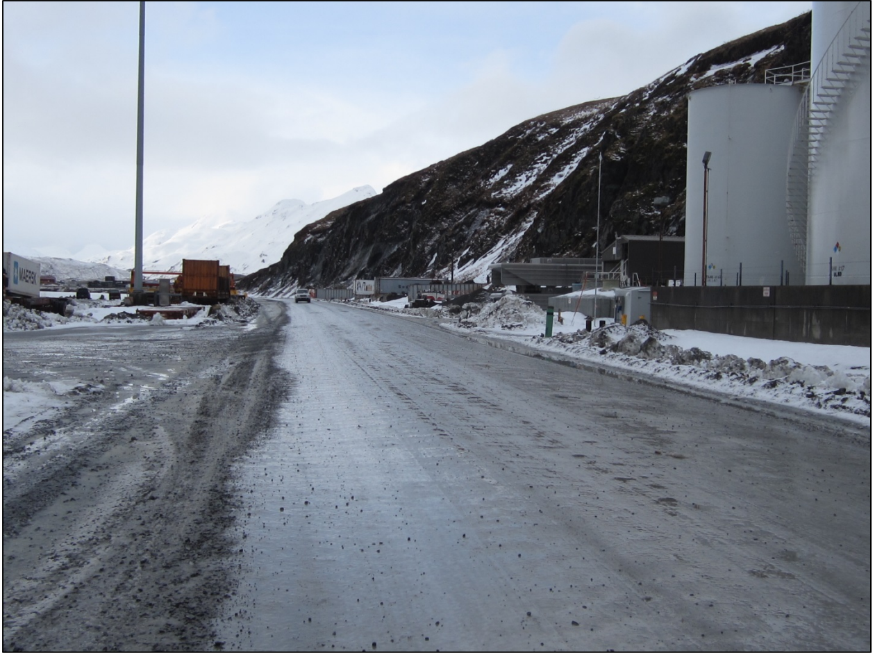
PHOTO 5. Ballyhoo Road along the UMC City Dock Backreach Area (looking SW).
