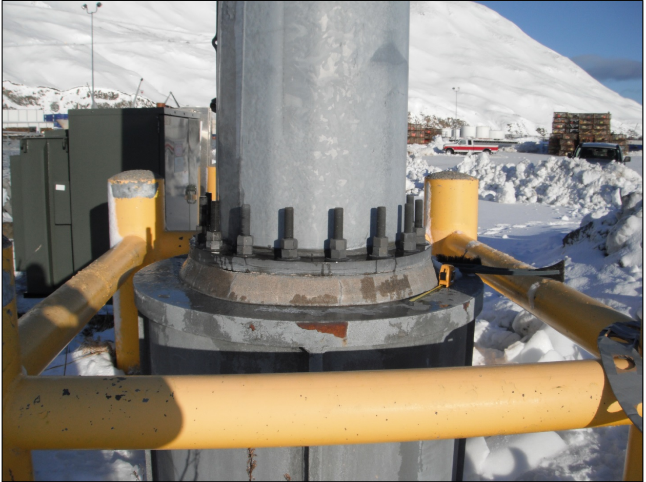
PHOTO 12. Base of South HML at Light Cargo Dock.
