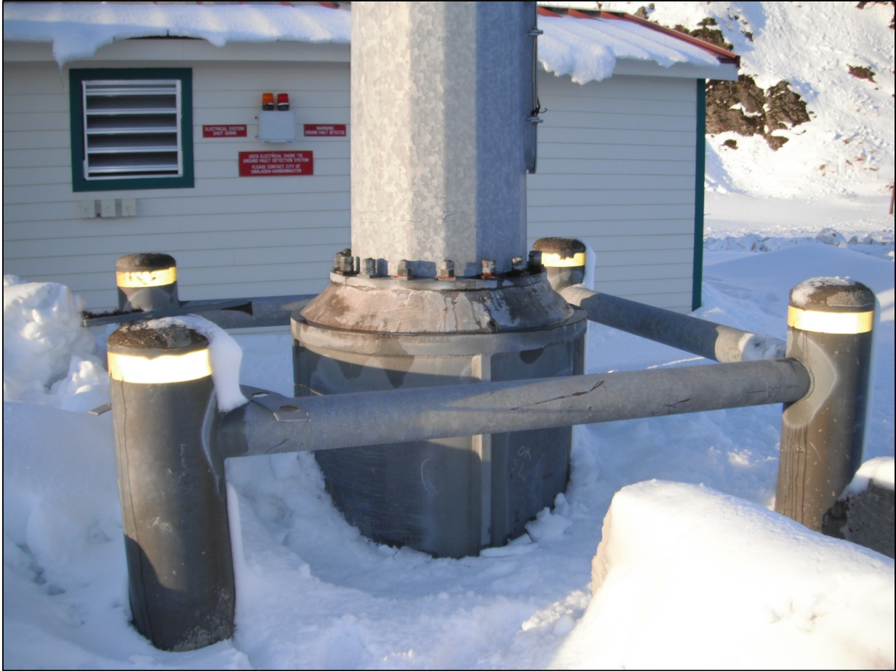
PHOTO 8. Base of North HML at UMC USCG Dock (looking N).
