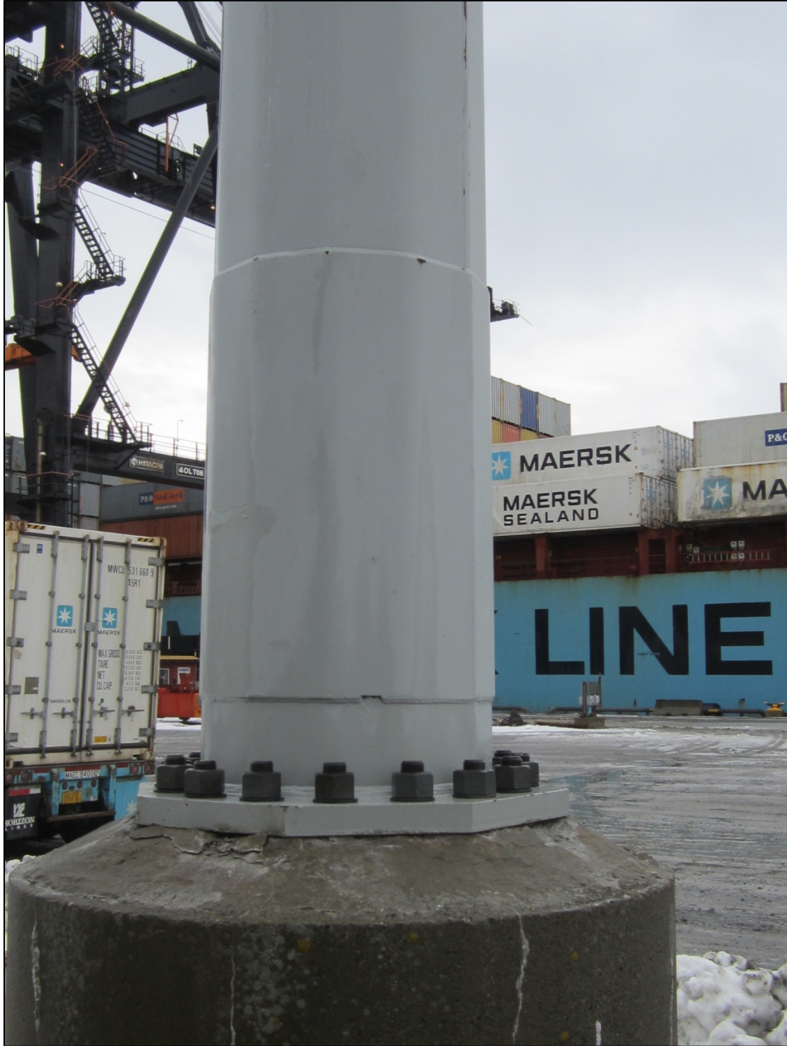
PHOTO 4. Base of North HML at UMC City Dock.
