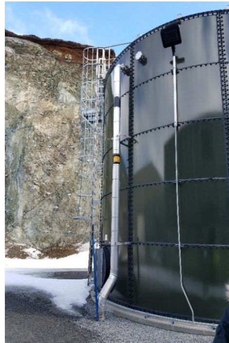
Figure 5-6. Sludge Holding Tank and Adjacent Bluff
