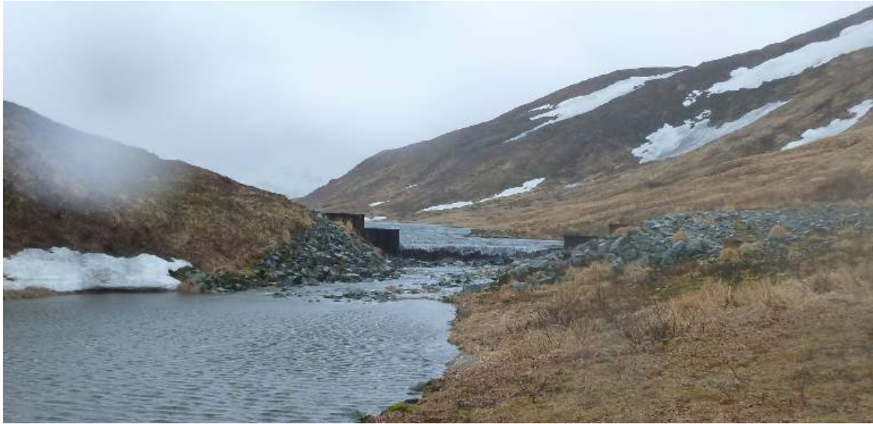
Figure 28: Icy Lake north sheet pile dam and spillway
