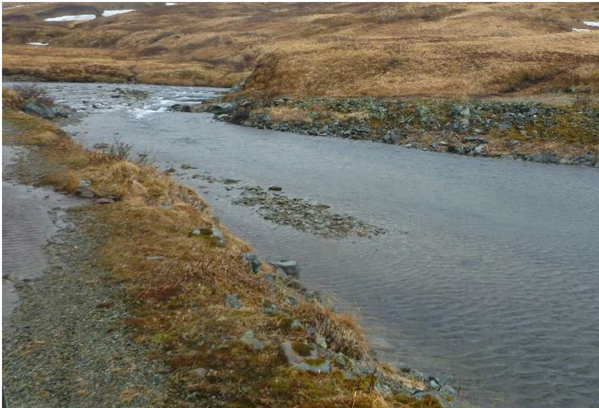
Figure 30: Gravel bar that has accumulated at inlet end of Icy Creek Reservoir
