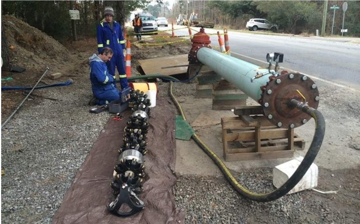
Figure 27: PICA Corporation See Snake and tool insertion port (image source www.picacorp.com )
