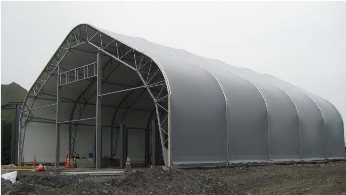
Figure 2. Sprung Fabric Structure
