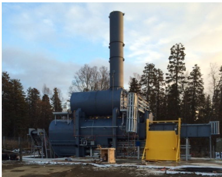
Installation of Gasification System, Dillingham, Alaska
