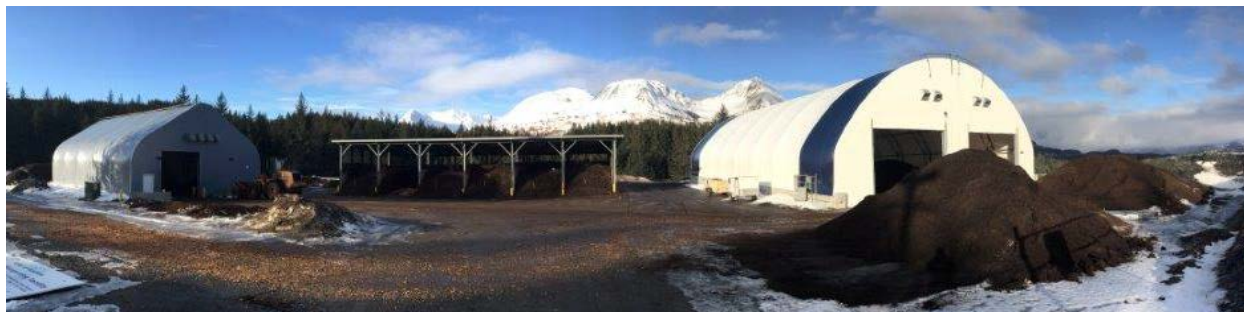
Biosolids Composting System, Kodiak, Alaska
