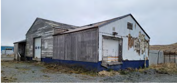
Figure 51. Naval Operating Transport Service Warehouse, facing northwest. (©TNSDS 2022)
