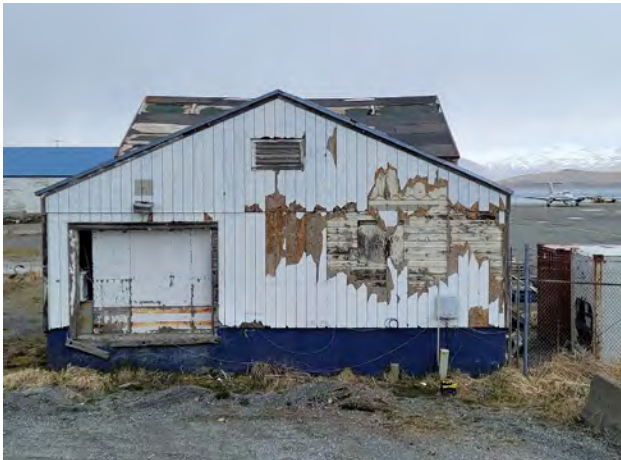
Figure 56. East facade of the Naval Operating Transport Service Warehouse (©TNSDS 2022).
