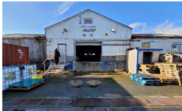
Figure 55. North facade of the Naval Operating Transport Service Warehouse (©TNSDS 2022).
