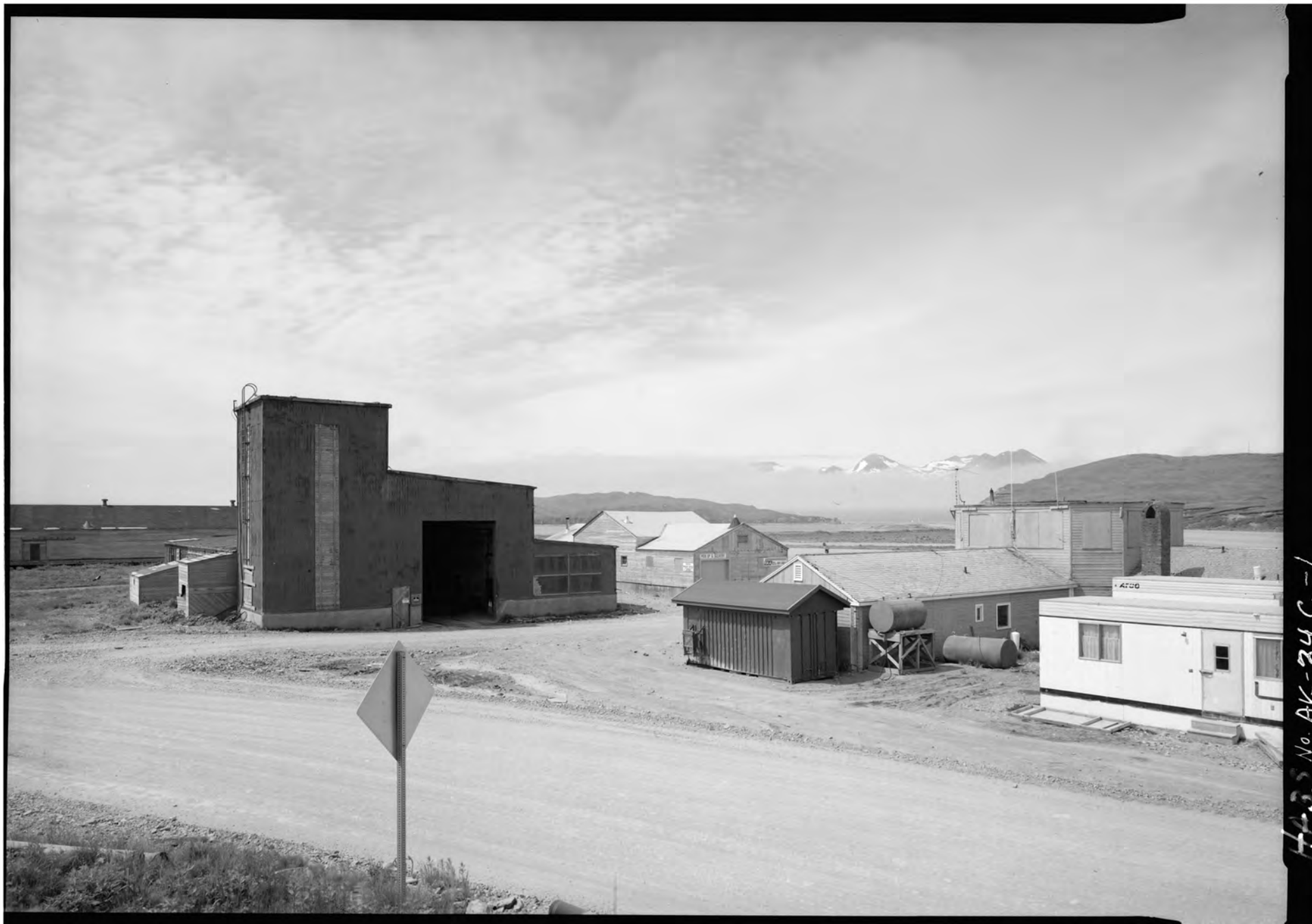
Attachment 3 - Photograph 1 : HABS No. AK-34 Record Documents, Survey Photograph HABS No. AK-34-C1 Facing northwest and starting left to right - Torpedo Bombsight and Utility Shop, Naval Operating Transport Service Warehouse (center background), Aerology Operations Building, and Trailers
