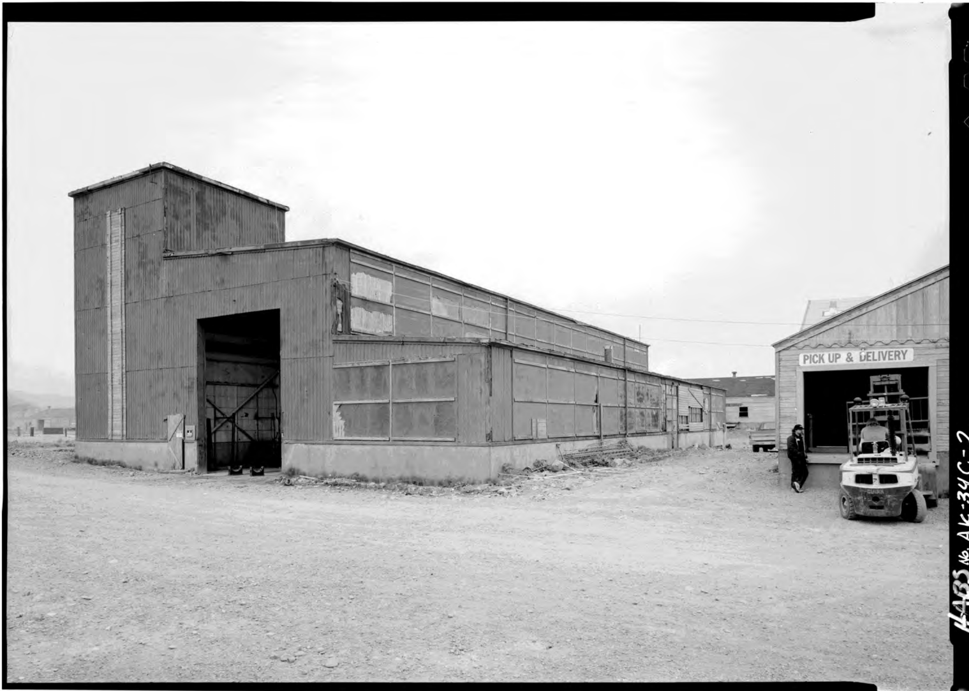
Attachment 3 - Photograph 3 : HABS No. AK-34 Record Documents, Survey Photograph HABS No. AK-34-C2 Facing west - Torpedo Bombsight and Utility Shop (left and) Naval Operating Transport Service Warehouse (right)
