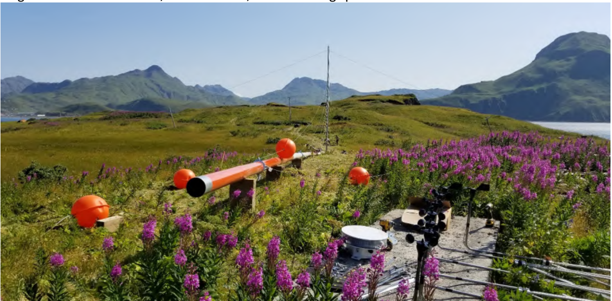
Hog Island tower during assembly, view south
