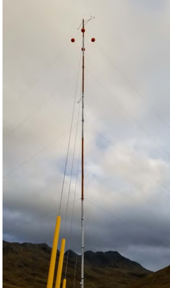
ICR 34 m, northwest side (view to southeast)
