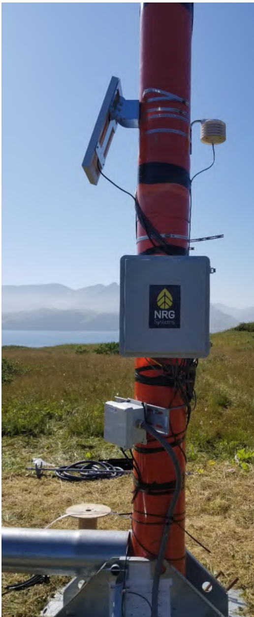
Hog Island 60 m, tower base
