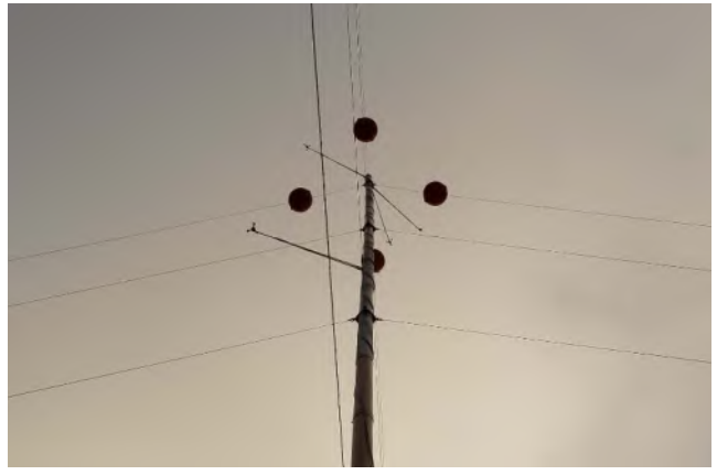
ICR 34 m, uptower, northeast face
