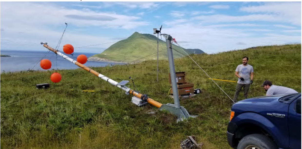
Bunker Hill 10 m met tower during installation
